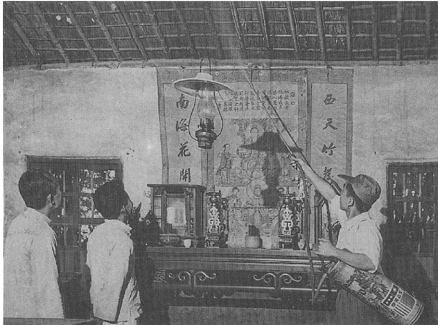
Fig. 51: Ceiling of a house being sprayed Source: JCRR
