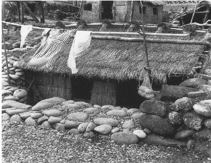
Fig. 92: A typical Typhoon-proof "winter house"
